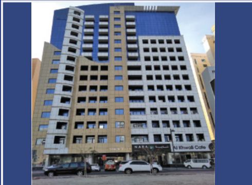
Dream Tower - Al Mamzar, Dubai MEP Annual Maintenance
