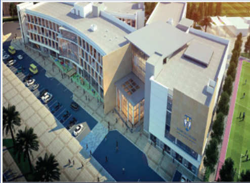
Bighton College - Al Barsha, Dubai Supply, Installation, Testing & Commissioning of HVAC System (VRV System)
