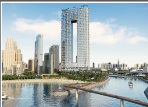
The Address Residences, Jumeirah Resort & Spa - Dubai Project Supplies: FAHUs, AHUs, AC FCUs
