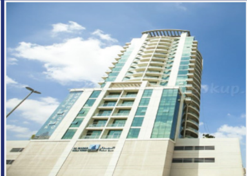
Scala Tower - Business Bay, Dubai MEP Annual Maintenance
