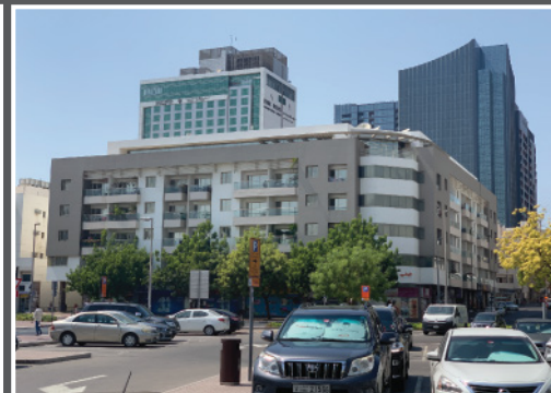
Talal - 7 Building - Karama, Dubai External Cladding & Painting
