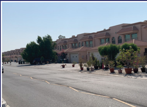
52 Villas - Dubai Real Estate - Al Safa, Dubai External Building Painting
