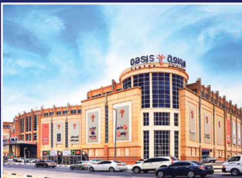
Oasis Mall - Al Quoz, Dubai Installation of Complete HVAC Systems
