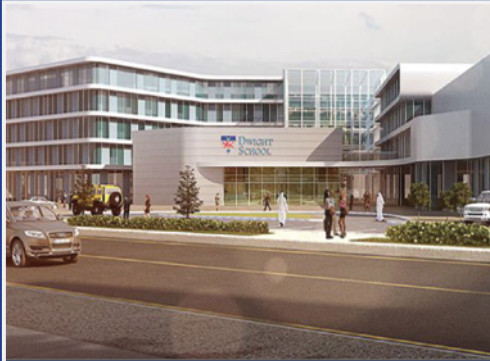
Dwight School - Al Barsha, Dubai Supply, Installation, Testing & Commissioning of HVAC System (VRV System)
