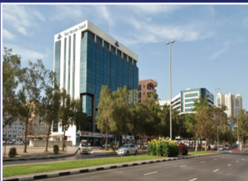
Rais Hassan Saadi Building - Bur Dubai Chilled Water Network & Retrofit Works
