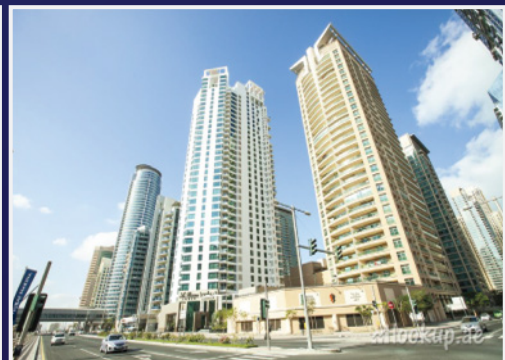
Marina Mansions - Dubai Marina, Dubai MEP Annual Maintenance
