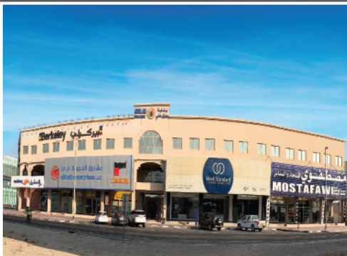
Jebel Ali Building - Al Quoz, Dubai Building Maintenance
