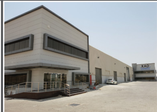
KAD Air Conditioning - Dubai Industrial City - Dubai Building Maintenance
