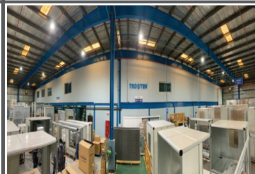
Trosten Industries Company LLC, Plant 2 - Mezzanine Floor for Offices Design & Build
