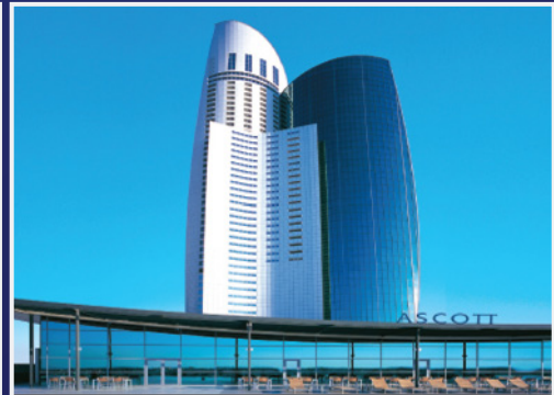
Ascott Park Place - Sheikh Zayed Road, Dubai MEP Annual Maintenance
