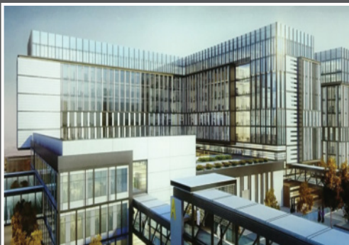
Fly Dubai New Headquarters - Dubai Project Supplies: Acoustic Liner and Aluminium Cladding Sheets
