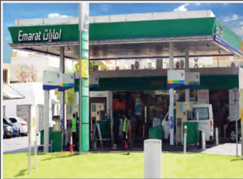
Emarat Service Stations - Multiple locations, Dubai
