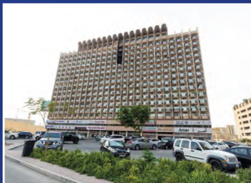
Sheikh Rashid Building - Al Karama, Dubai
