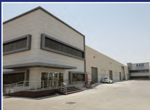
KAD Air Conditioning - Dubai Industrial City - Dubai
