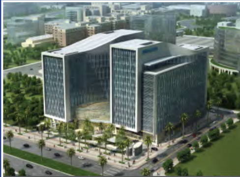
Parsons Regional HQ - Abu Dhabi
